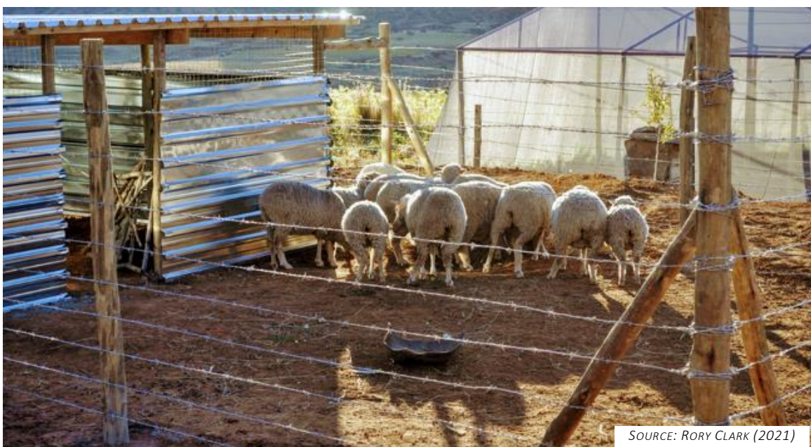
FIGURE 37: NEWLY CONSTRUCTED SHEEP RUN
